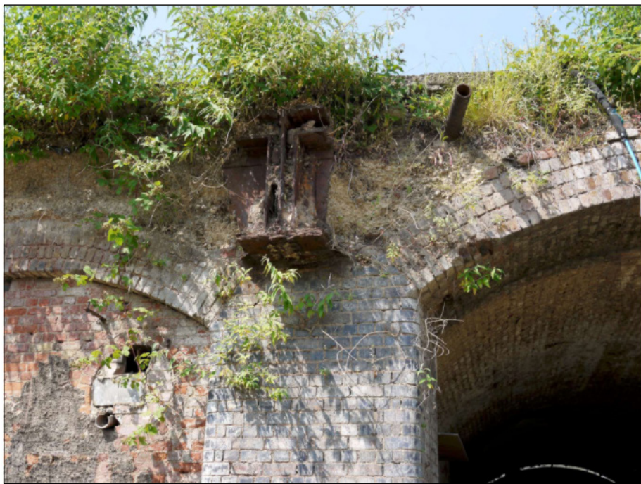
REPAIRS TO BRICKWORK - This work will include vegetation removal, repointing and replacement of badly spalled or missing bricks.
